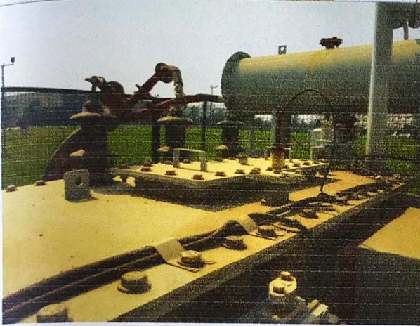
HT termination of Transformer is not done properly. Terminals are under stress. Proper contact area is not established. Bent Insulator metallic rods.
