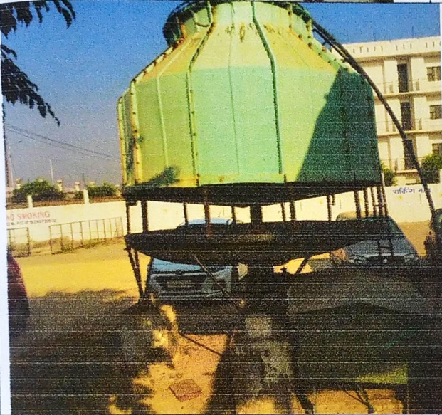
Cooling Tower not maintained
